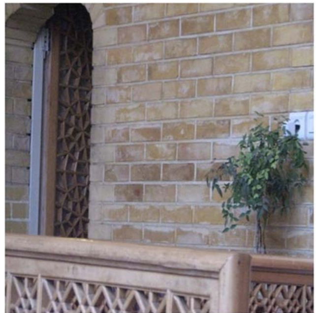
Figure 11. The brick work of wall of Eastern room (Madar).
