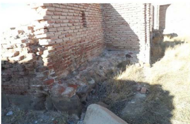
Figure 6. Walls were made of brick and stone foundation (Authors).
